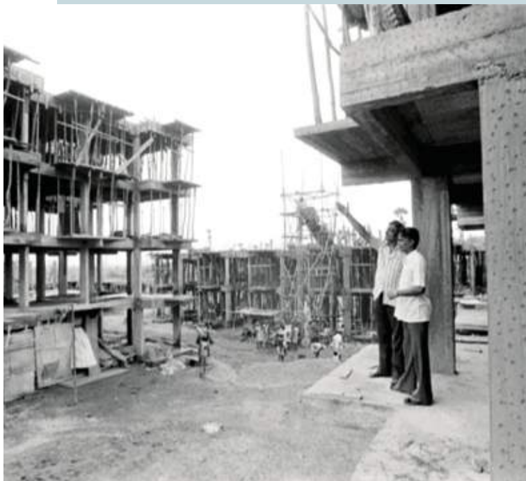
India: HDFC-financed housing units under construction, 1980.
